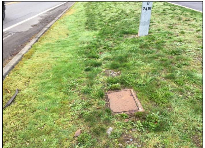
Electrical box indicates utility conflicts may be present.
