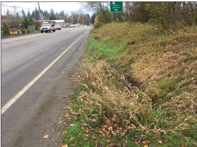
Ditch in ROW looking north.
