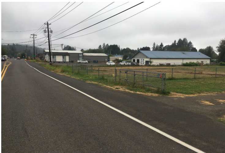
Proposed retrofit location looking south.
