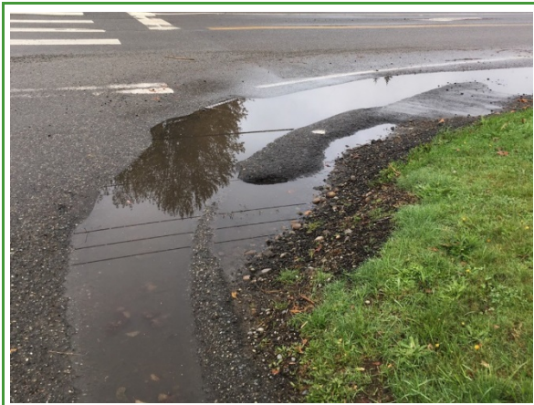
Drainage from Impervious Surface
