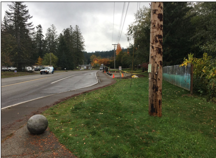
Proposed retrofit location looking east.
