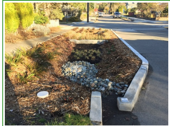
Example Bioretention Design
