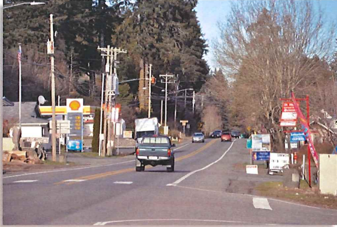
SR 3 looking north at Evans Street
