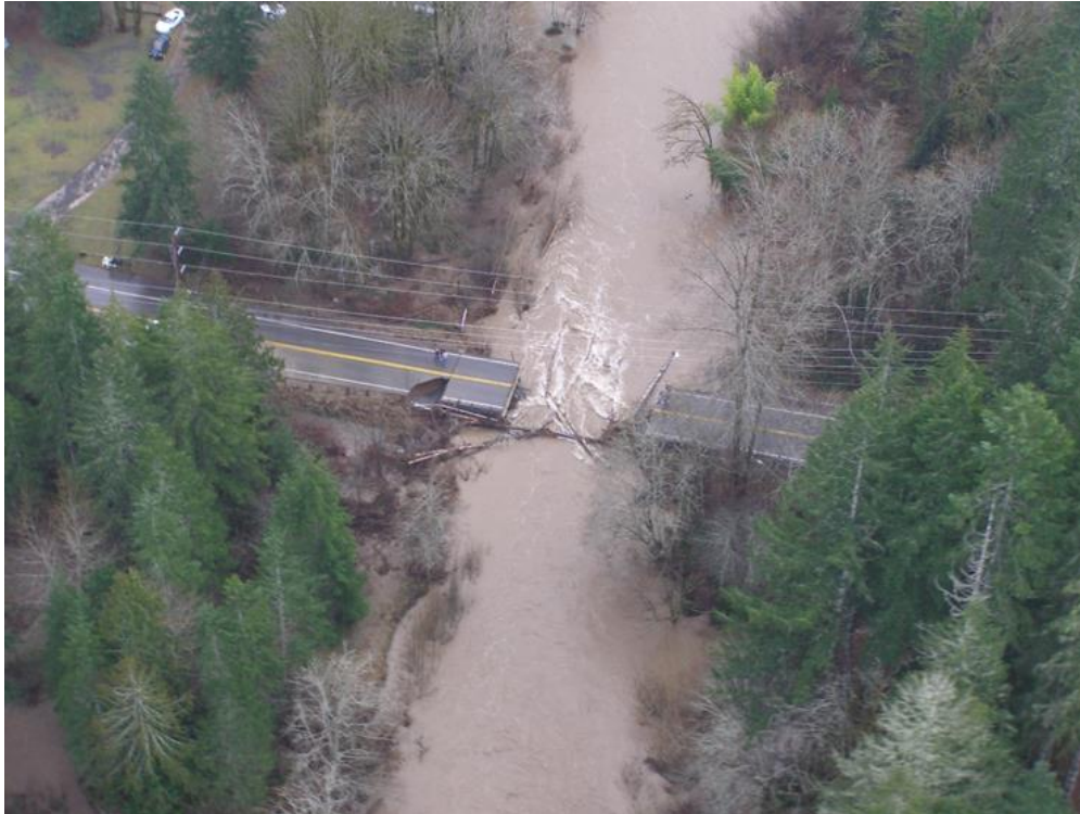
Figure 7-9 Belfair-Tahuya Bridge on the Tahuya River December 2007 (DR 1734)
