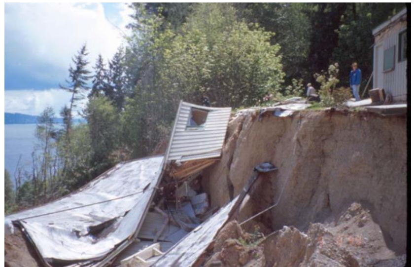
Figure 8-6 House destroyed by landslide in Lilliwaup Winter 1998-1999
