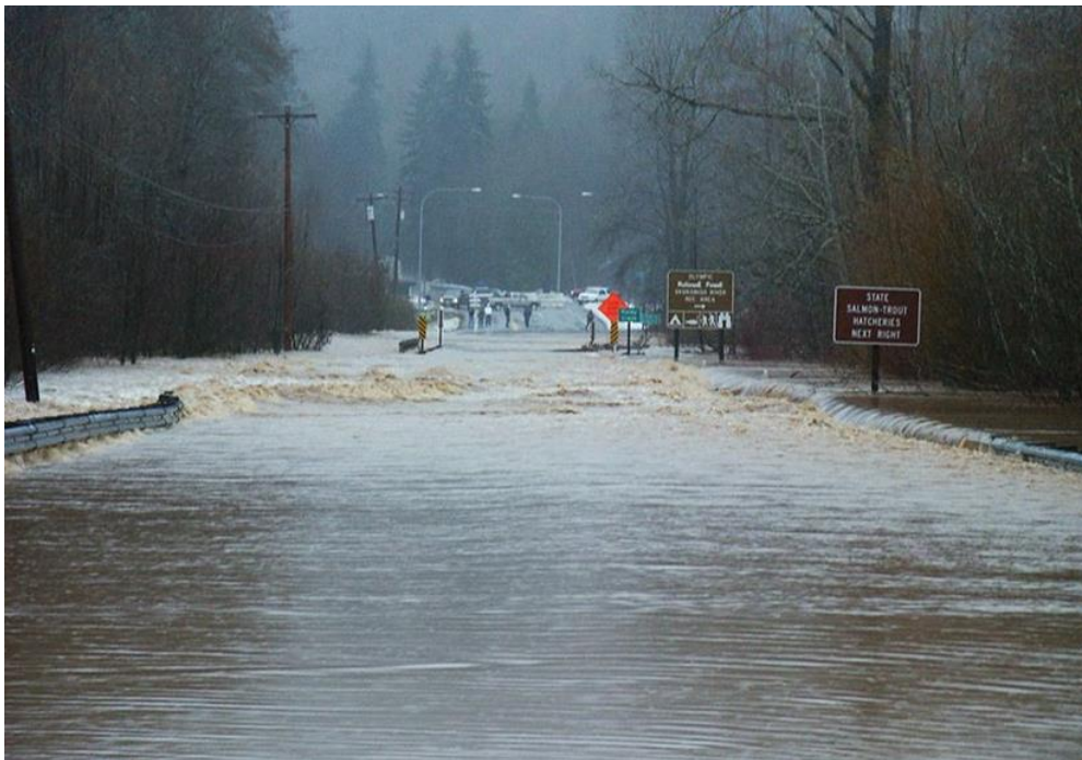
Figure 7-8 December 3, 2007 Incident Highway 101 North of Shelton
