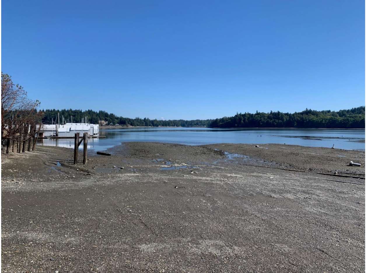
Figure 1: Photograph of existing boat launch at the Oakland Bay Marina. The gravel boat launch ends at +10 MLLW, and below that the substrate is too soft to launch boats.
