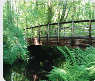
Decker Creek Bridge
