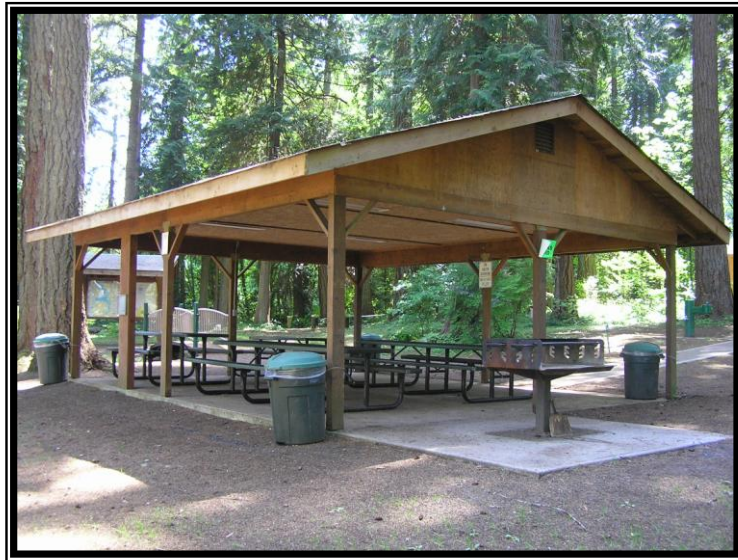
WALKER PARK GROUP PICNIC SHELTER
